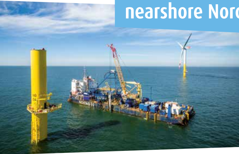
Installation of cables on the Nordergründe construction site
